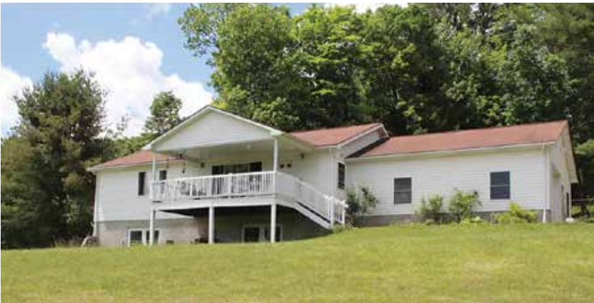
The facilities director's house was built in 1998 and includes a basement apartment.
