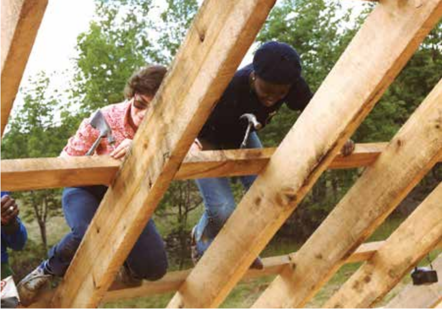
Janet Landis, Jackie Buck, nailing purlins.
