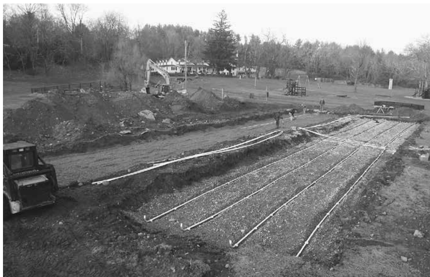
The sewer system is expanded in December 2012 to accommodate Promise Woods.
