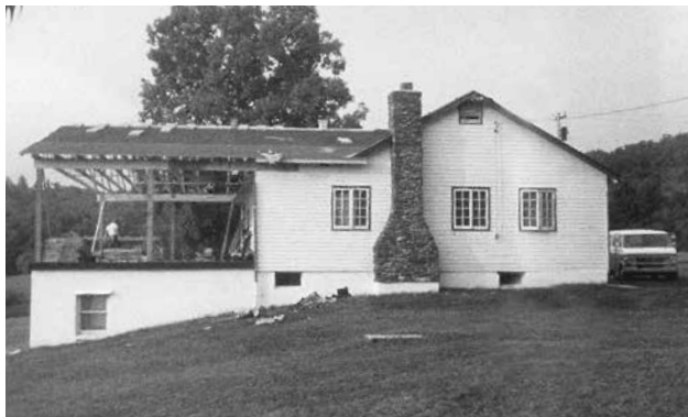
Chapel porch receives a roof, 1984.
