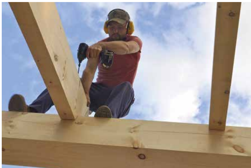
Kenton Baer fastens rafter to beam of Promise Woods cabin.
