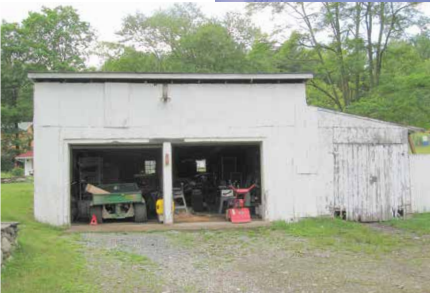
Garage: first building project undertaken by Camp Deepark was constructed with salvage materials from barn removal.
