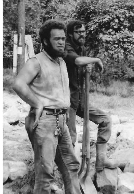
Maynard Shirk, left, and Lowell Jantzi survey construction of cabins on the hill, 1975.
