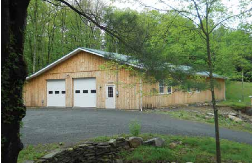
The maintenance building was constructed in 2009 and includes offices, mechanical shop, wood shop, and storage.
